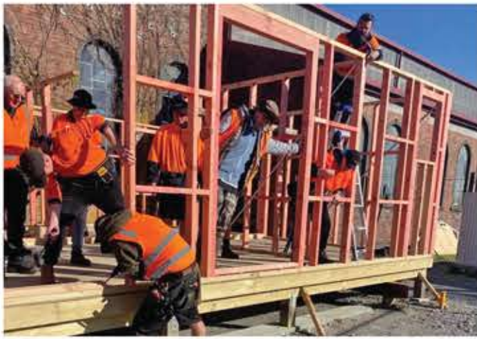
Polytechnic Carpentry students frame the 2021 Project House.
